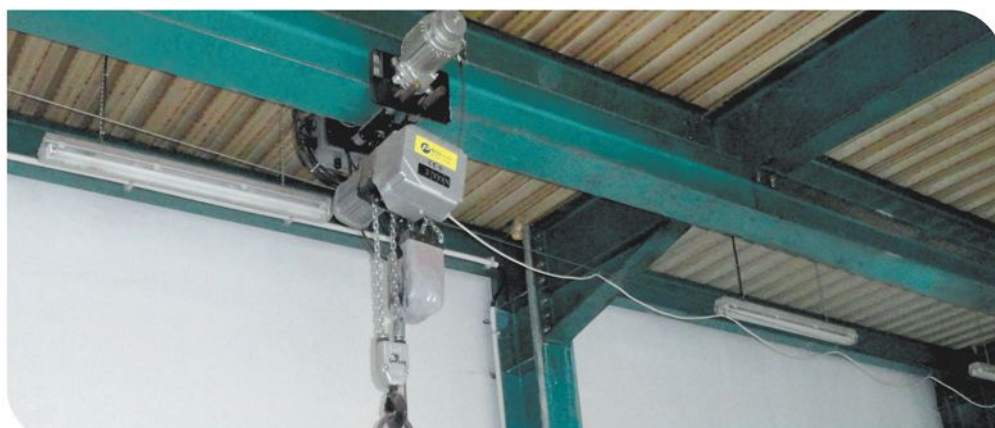
PRO-CV trolley fitted with PRO-CTS electric chain hoist
